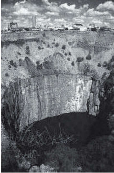
Figure 1.19: The Big Hole, Kimberley, South Africa: the world's first open-pit mine of modern proportions, albeit largely excavated before the advent of large-scale earth-moving equipment. The cylindrical shape of the Hole reflects the form of the igneous intrusion which hosted the diamonds. The total depth, at 215 m, is belied by the partially flooded state of the void at present. The void forms a 'through flow' pit lake (see Figure 3.42a; Section 3.11.1). (Photo: Kimberley Mine Museum).
