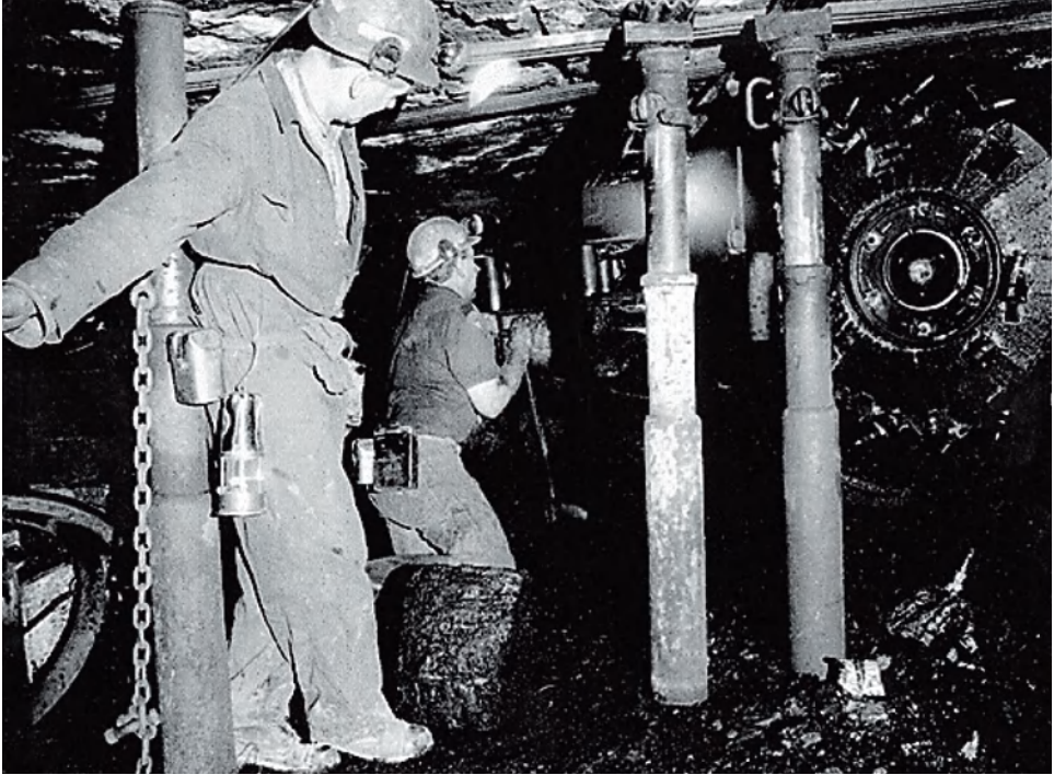
Figure 1.14: Close-up view of a longwall coal face, showing the drum shearer (circular feature on the right) which is being adjusted by the miner working within hydraulic supports. In the foreground is the Deputy (supervisor) with a flame lamp at the ready to check for gas, for the working face is generally the most prolific source of methane in a working coal mines. (Photo: A. Doyle).
