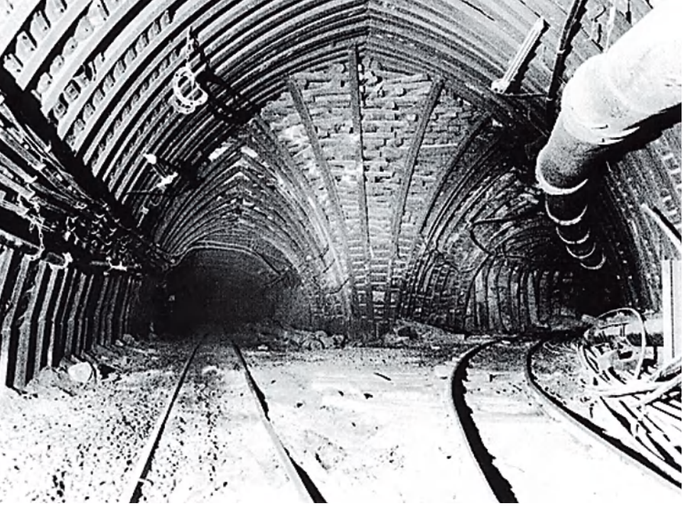
Figure 1.8: Example of a major deep mine “level”, in this case a junction of two main locomotive roadways in a deep coal mine (Westoe, north-east England). This locality (known as “Cathedral Junction”) is the point at which the access from the foot of the main shaft diverges towards the two principal working districts in the mine. The roof support is engineered for permanence: steel arch girders with intervening steel cross-plates. The large pipe entering the right-hand branch of the level at head-height carries compressed air for ventilation. Most of the other continuous “pipes” in this view are electricity cables, with the exception of two pipe ranges conveying pumped mine water: the lowermost narrow pipe, hanging on chains on the left-hand wall, serves a local pump, whereas the large pipe at floor level on the right (partly obscured by spare materials) is a major pipe-range from the working districts. (Photo: A. Doyle).
