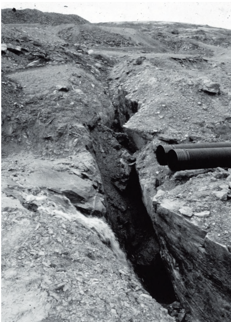
Figure 1.34: A stream cascading into an open stope which has been driven (probably unintentionally) all the way to daylight. The scene is at an abandoned base metal sulphide mine in central Norway. (Photo: D. Banks).
