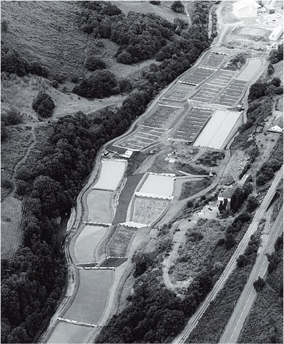
Figure 5.1: An extreme example of the large land take a passive mine water treatment system can demand: the UK Coal Authority's Taff Merthyr aerobic wetland system; South Wales. The photograph was taken shortly after commissioning of the system in the year 2000. Mine water emerges at surface from an old mine shaft in the center of the treatment area. It is then cascade-aerated and split three-ways, into each of three conspicuous sedimentation ponds, each of which is followed by a series of aerobic wetlands. The size of the system in this case made a major contribution to the clean-up of derelict land associated with the former colliery, and is integrated with a newly-established country park and adjoining commercial premises. (Photo: UK Coal Authority).
