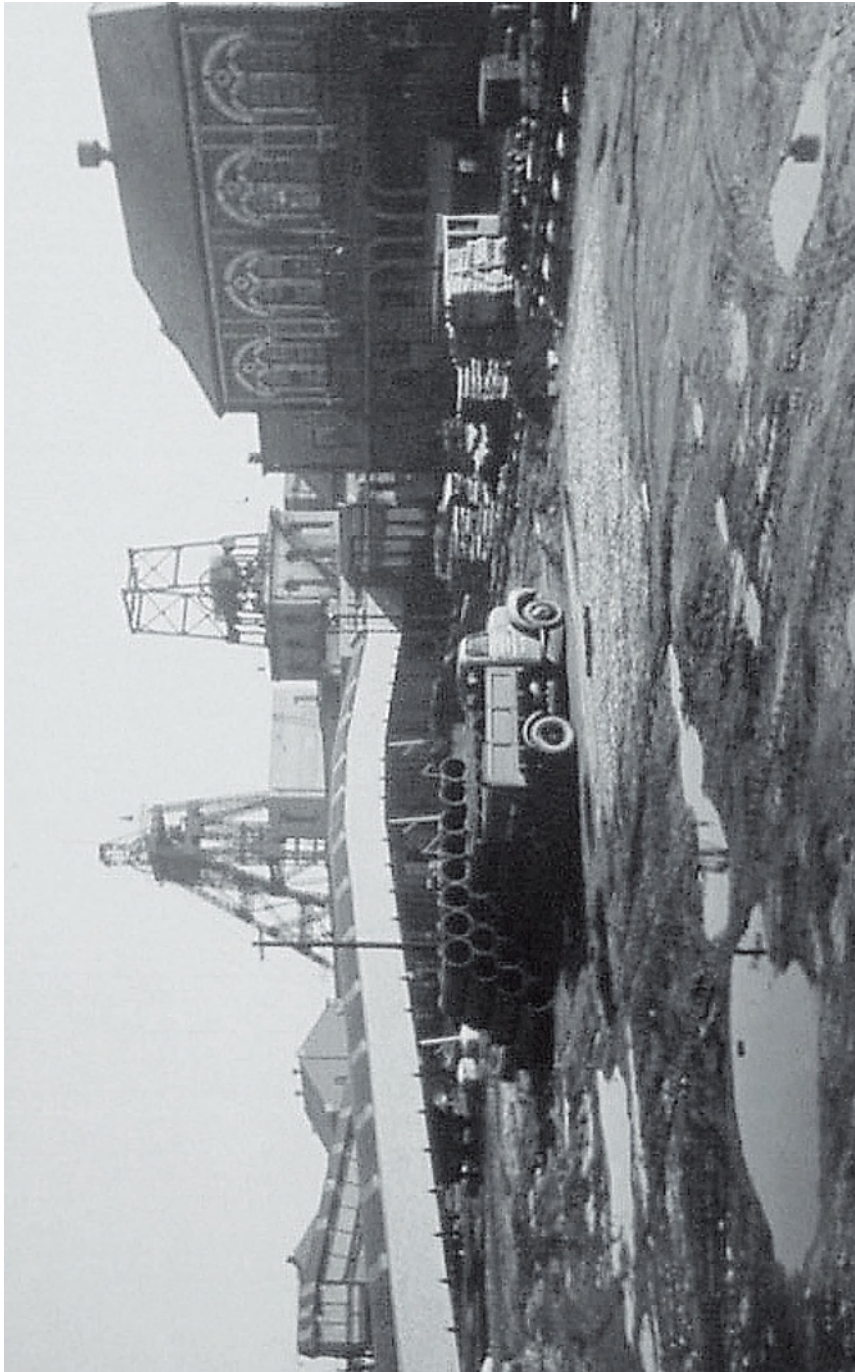
Figure 1.3: A typical pit-head scene, in this case at Boldon Colliery, Durham (UK), in 1950, showing two closely adjoining shafts, marked by the two headframes. The twin shafts provide between them a complete ventilation circuit for the mine and two independent means of egress from the underground workings. (Photo: National Coal Board, salvaged by A. Doyle).
