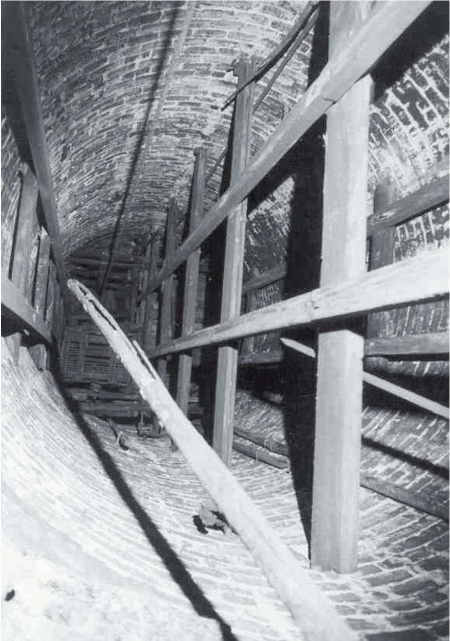
Figure 1.7: A view up a typical staple shaft in an underground coal mine in the Great Northern Coalfield (UK). The landing of the next highest mine level can be clearly seen. The timber work partitions the shaft for different uses (occasional haulage in the central sector, and pipe ranges and power lines in the sector behind the timber framework on the right). (Photo: A. Doyle).
