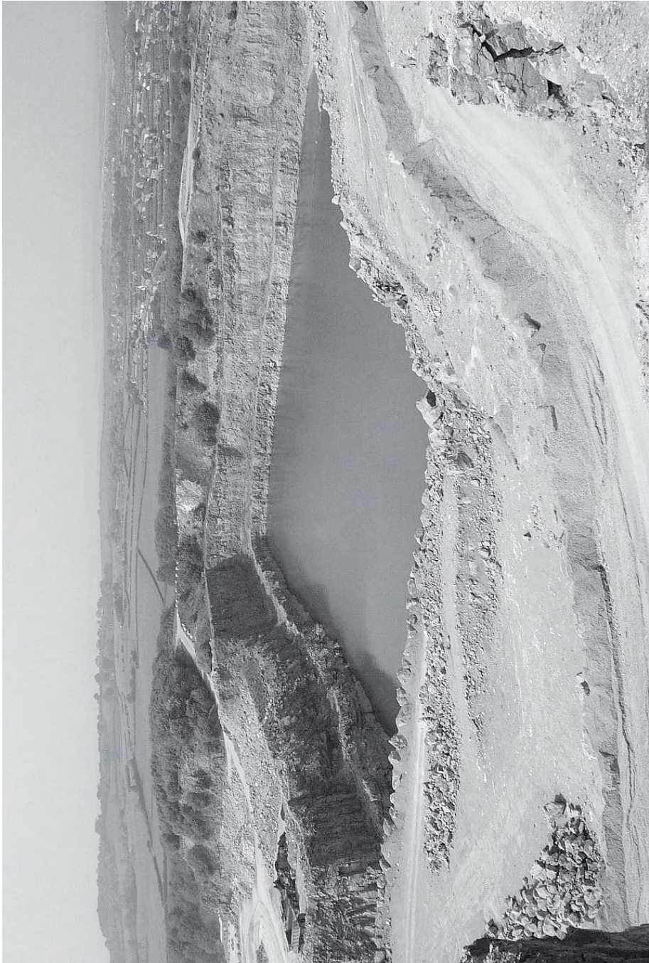
Figure 3.27: A major sump in a surface mine: a limestone quarry in NW England.
